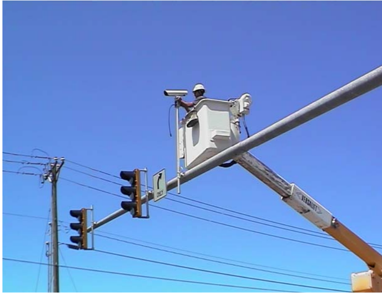
Photograph 3 Camera Installation, Route 229, Southbound, Southington, CT
