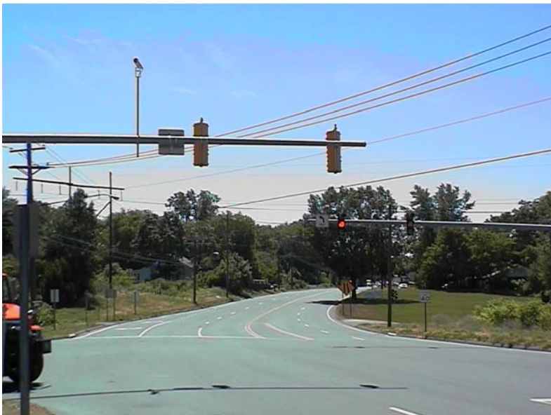
Photograph 4 Route 229, Southbound, Southington, CT
