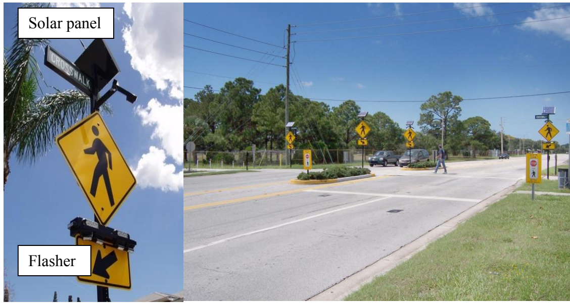
2 FIGURE 1 RRFB close-up and system installation at the Pinellas Trail crossing and 3 22 nd Avenue N.
