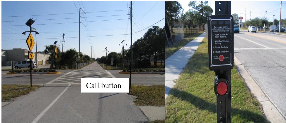
1 2 FIGURE 2 RRFB system and close-up view of call button at the Pinellas Trail 3 crossing.
