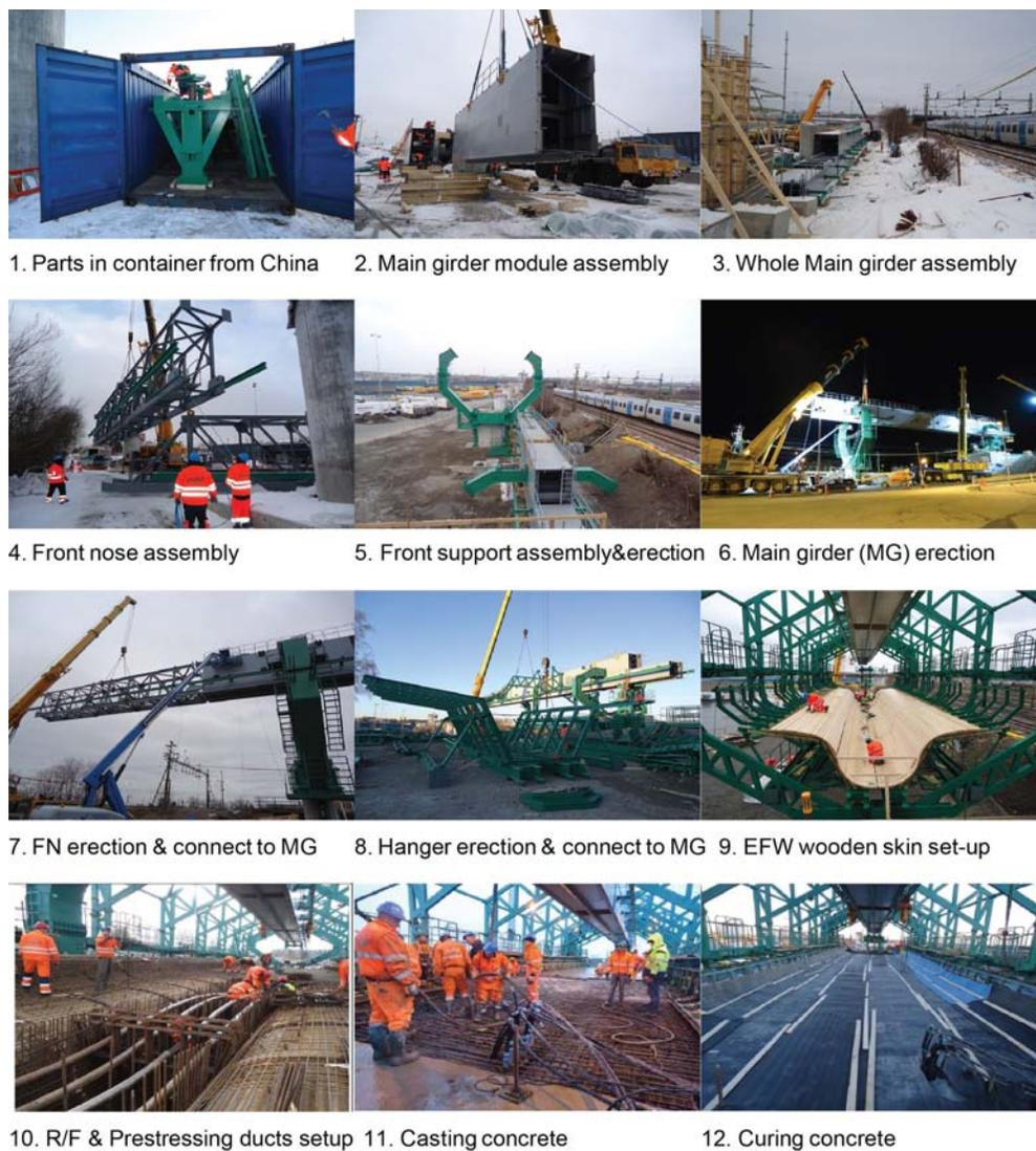
Fig. 6 Assembling and erecting sequence of the SL-MSS
