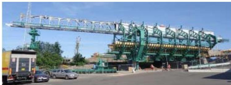
Fig. 8 The MSS in concreting position for start span during August 2012
