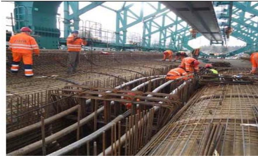
Fig. 7 Reinforcement and prestressing steels installation
