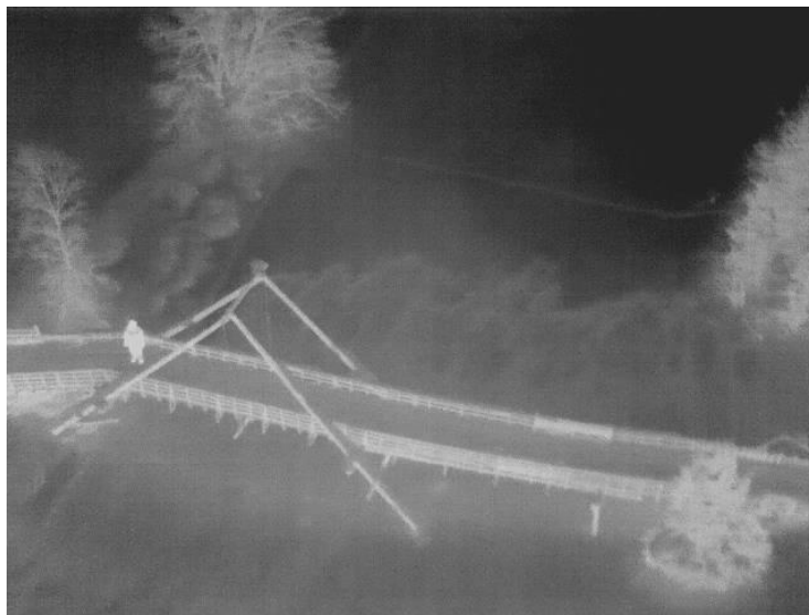
FIGURE 3 Infrared-red bridge photo
