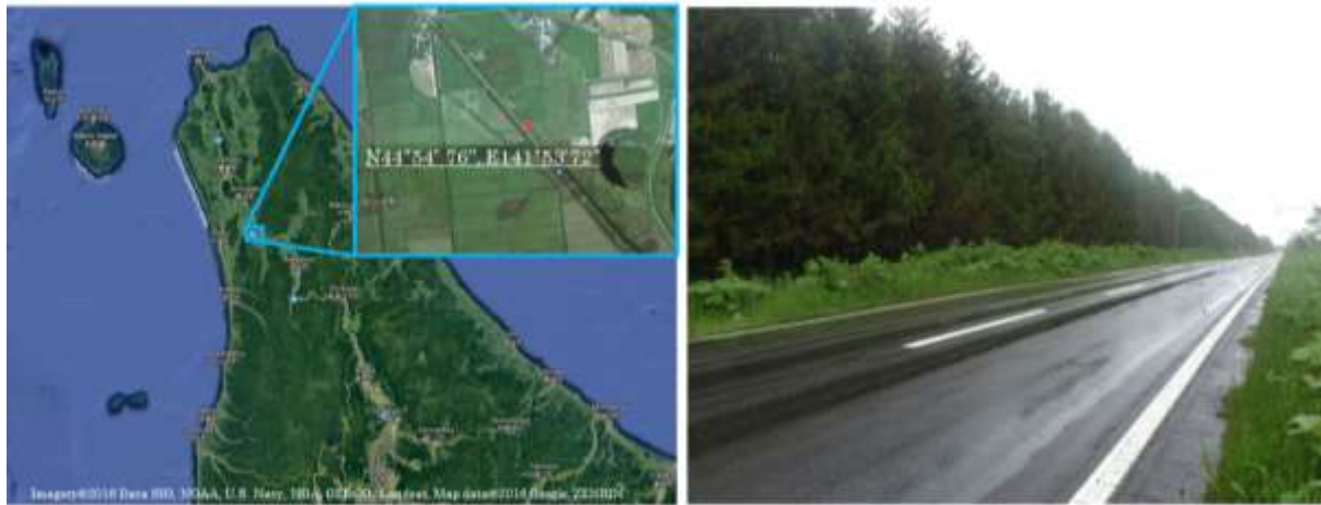
1 2 FIGURE 7 LSF site at N44^{\circ}54'76'' , E141^{\circ}53'72'' (left), and a picture of National Route 40 at the 3 observation point (right).
